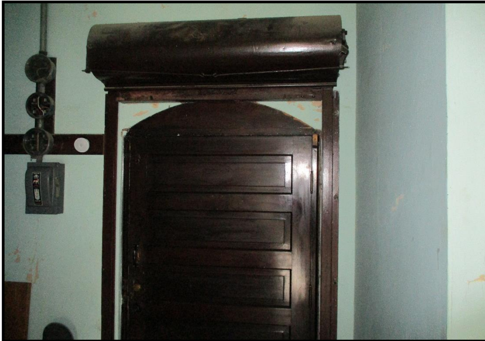
Doorway to Adjacent Building
